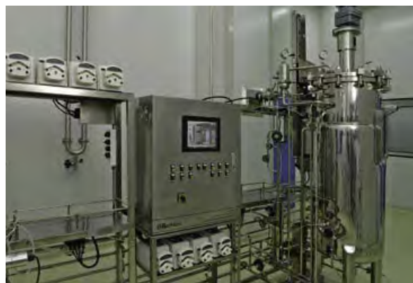
Fermentation Control System
